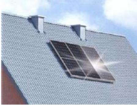
Fig14: A photovoltaic module with anti-reflective (AR) solar glass coating.<sup>2</sup>
