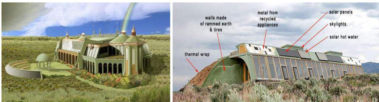
Fig. 13 Earthships are sustainable homes made of recycled materials, designed to integrate with nature as an example of biomimicry in the Ecosystem level
