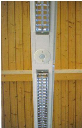
**Fig.7 lighting system is fitted with two sensors (occupancy sensors & light-level sensors)**
