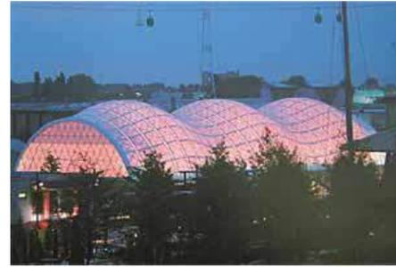
Fig.1 use a curvy paper tunnel supported by a matrix of recycled paper tubes to construct the "Japan pavilion" in "Hanover" exhibition in Germany ([http://www.designboom.com/history/ban\\_expo.html](http://www.designboom.com/history/ban_expo.html))
