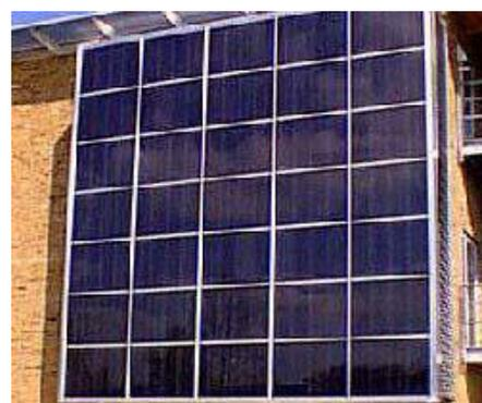
Fig.9 photovoltaic (PV) cells that produced a peak output of 1.5kW
