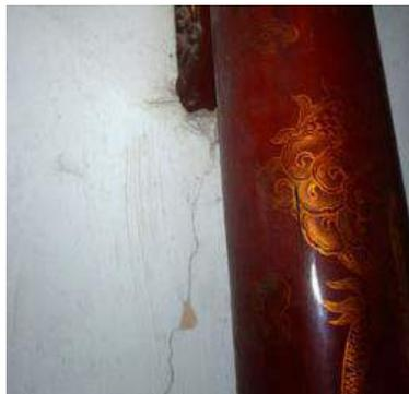
**Fig.6: Cracks resulting from failure of newly built walls.** (Source: Author)
