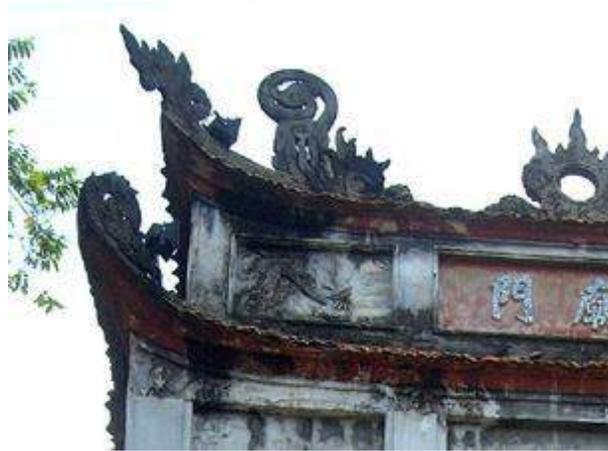
**Fig.5: Mould growth and deterioration of the temple.** (Source: Author)
