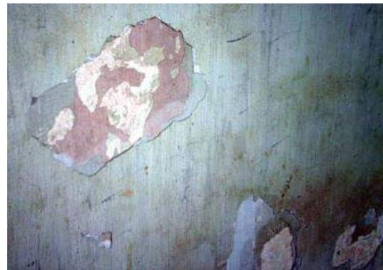
**Fig.7: Peeling of paint in walls renovated in 2001 due to the high humidity levels.** (Source: Author)
